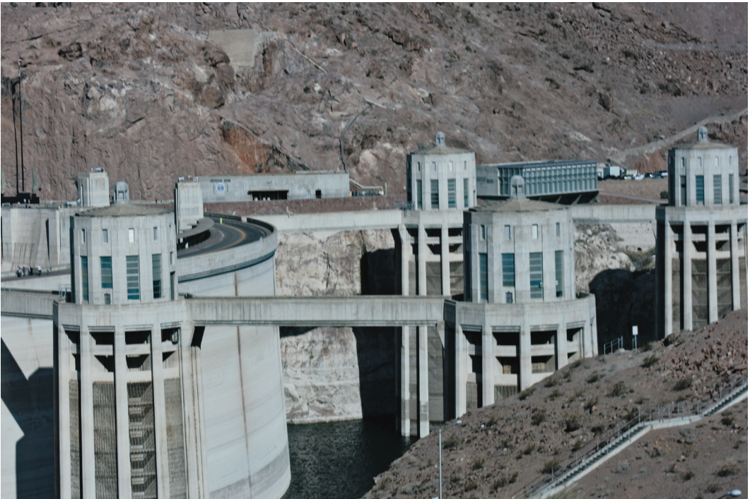
Figure 1.6 Hoover Dam is a concrete arch-gravity dam in the Black Canyon of the Colorado River, on the border between the states of Nevada and Arizona. It was constructed during the Great Depression and was dedicated on September 30, 1935 by President Franklin D. Roosevelt.
