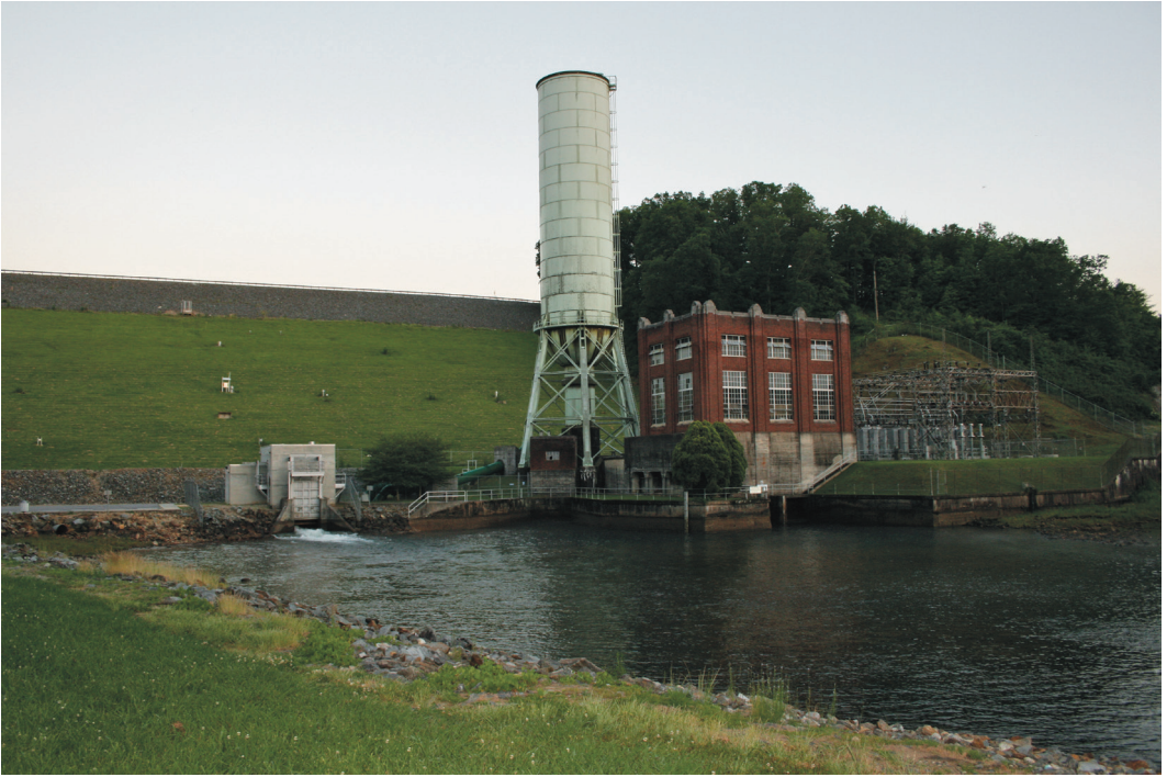
Figure 1.8 A Tennessee Valley Authority dam completed in 1930 in Blairsville, Georgia.
