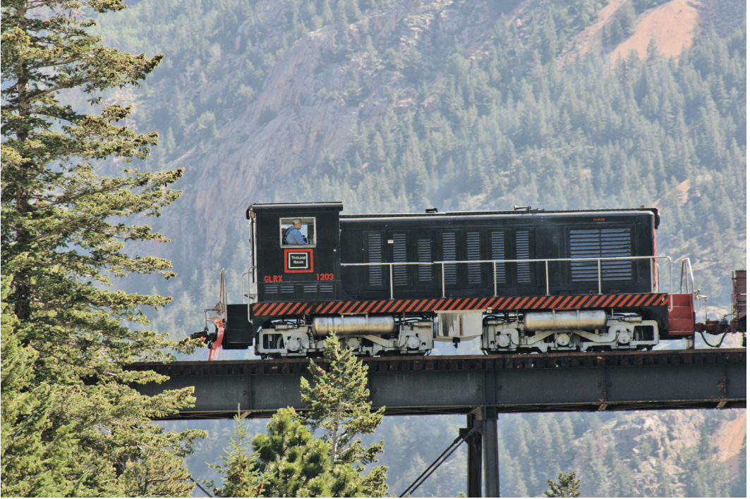
Figure 1.3 A railroad bridge built in Georgetown, Colorado, in the 1880s.
