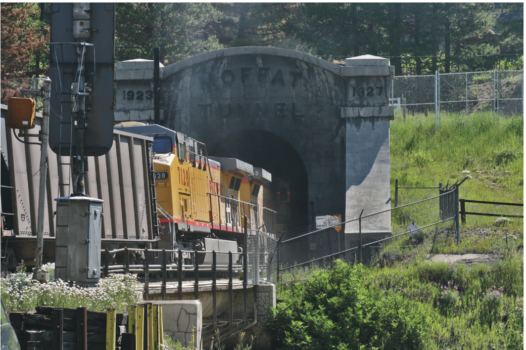
Figure 1.4 Railroad tunnel located in Winter Park, Colorado—constructed in 1927.
