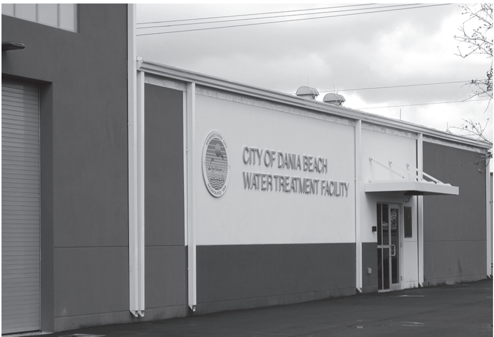
Figure 2 City of Dania Beach, FL LEED Gold nanofiltration water treatment plant
