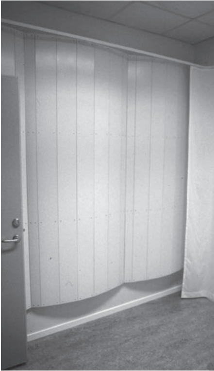
Figure 6.17 An example of a combination of slit absorber and diffuser for broadband control of the acoustical conditions in a recording studio in the Gothenburg Opera, Sweden. (Photo by Mendel Kleiner.)
