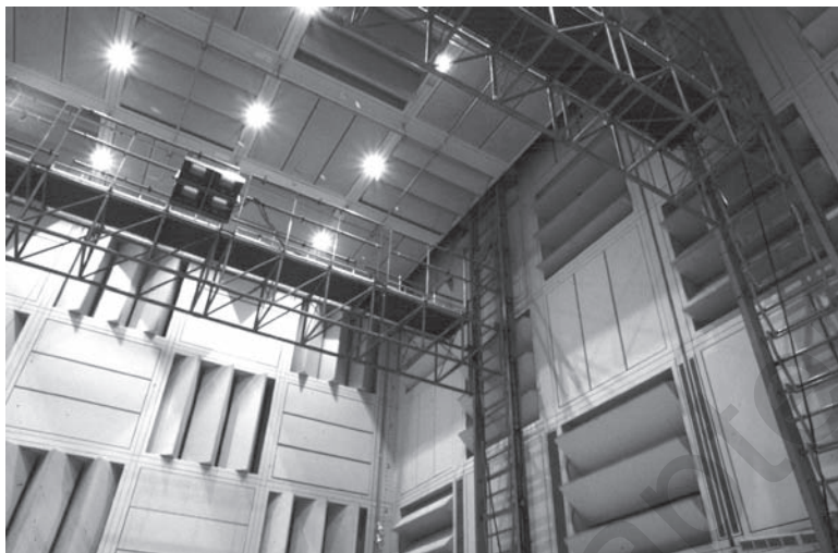
Figure 6.8 In this computer-controlled auditorium at IRCAM, Paris, the room acoustic conditions could be changed drastically using rotating wall sections. The sections were designed to be used as reflectors, scatterers, or absorbers (photo by Leif Rydén).
