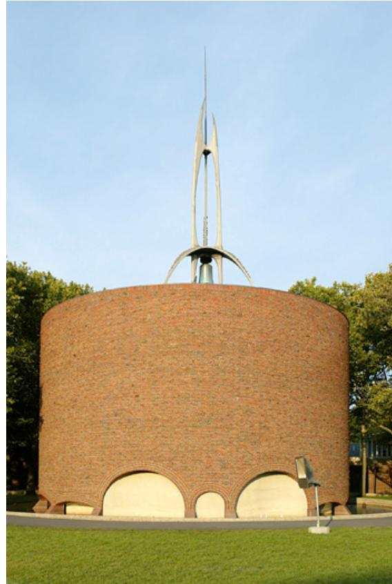
**Figure 1: Chapel Exterior** A moat surrounds the circular, drum-like building, and glass reveals surrounding the interior allow light reflected from the water to penetrate the interior. Architects; Eero Saarinen and Associates. Acoustics: Richard Bolt and Bob Newman, with assistance by William Cavanaugh, W. Ranger Farrell, and Jack Purcell. Photo by Morten M. Lund.
