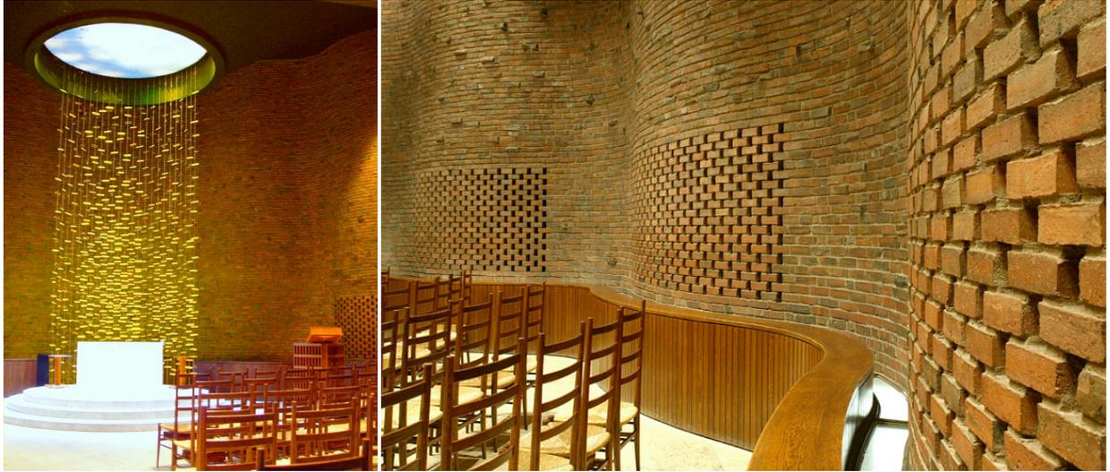
**Figure 2: The Chapel Interior, Left: View of the Serpentine,** Photo by Daderot at Wikipedia modified by D. L. Klepper. **Right:** Note two acoustical features: the undulations of the walls and openings in the brick wall, behind which is a 50mm glass fiber sound-absorbing treatment.
